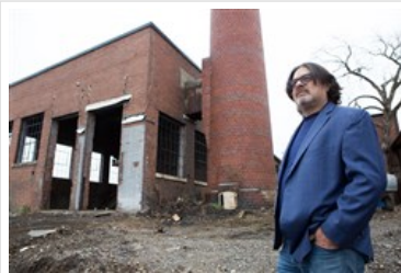
Tamay Ozari is in the process of redeveloping this old equipment warehouse he owns on Charlotte Ave. -- Michelle Morrow | The Ledger
